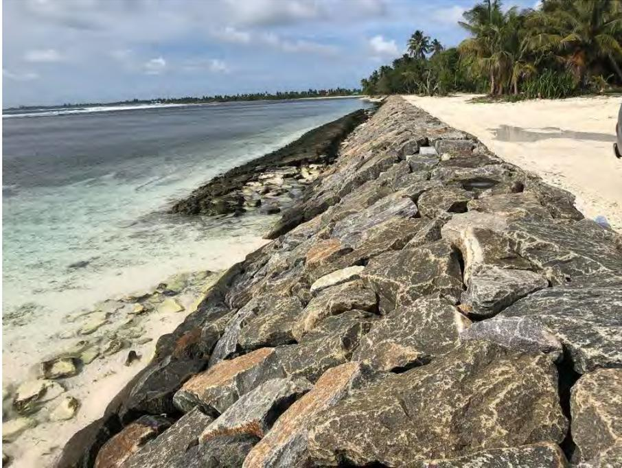
Figure 5. Rock Revetment Example
