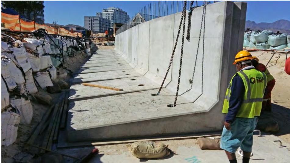
Figure 11. Precast Concrete Seawall Example
