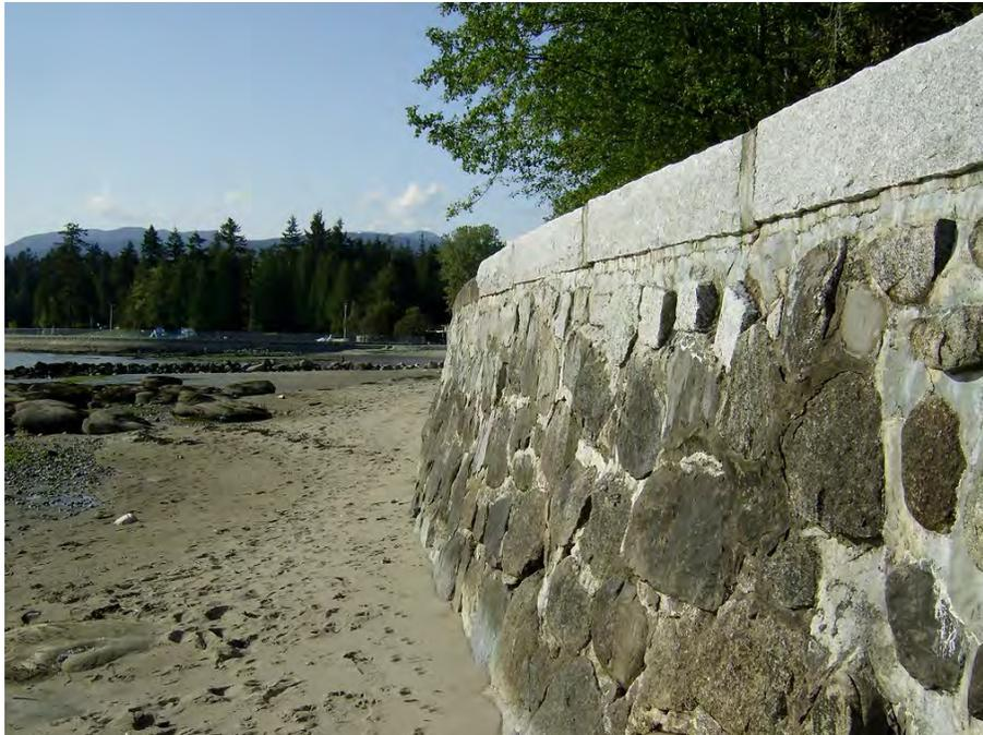
Figure 9. CRM Seawall Example
