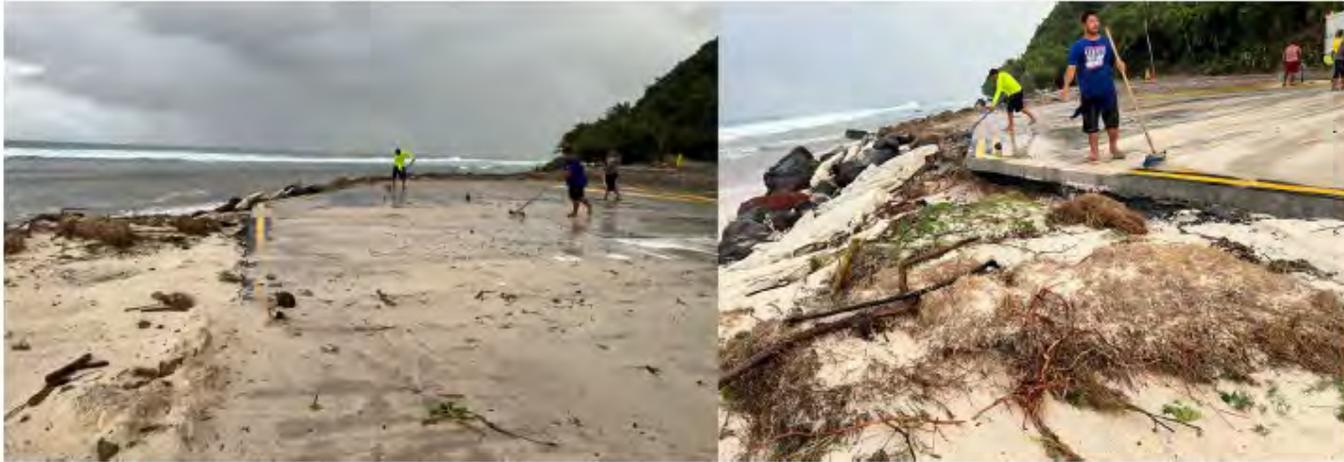
Figure 5: Erosion at New Runway. King tides and large swells combined to impact the newly constructed runway in July of 2022.
