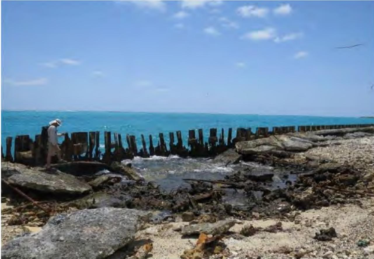
*Figure 8: Midway Atoll Sheetpile Seawall.* Photograph showing degradation of the sheetpile seawall at Midway Atoll. Photo by USFWS.
