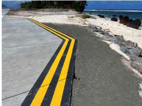
Photo 11. July 30, 2022, view to the southeast following repairs, showing extension of rock barrier and unpaved apron.
